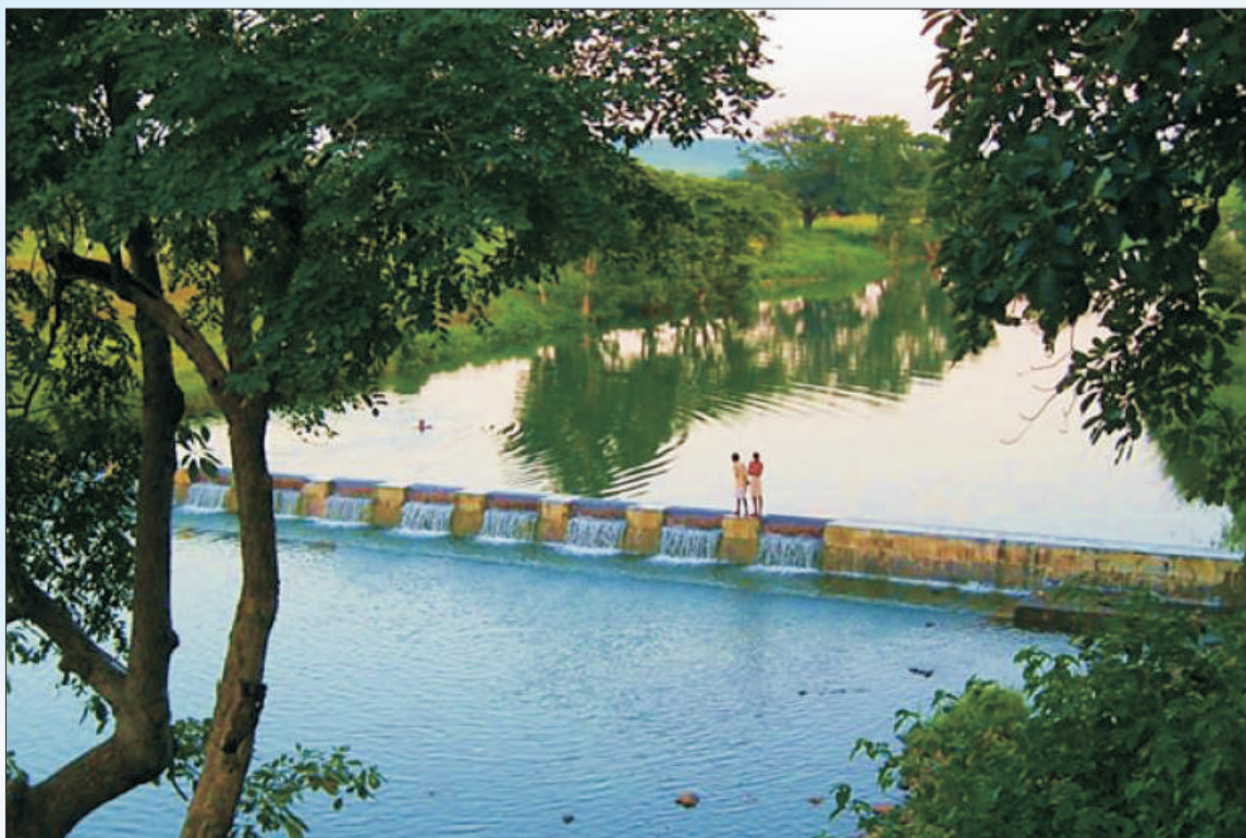
Anicut Constructed for Harvesting Water Under Watershed Project, Pratapgarh (Raj.) under IFFDC
